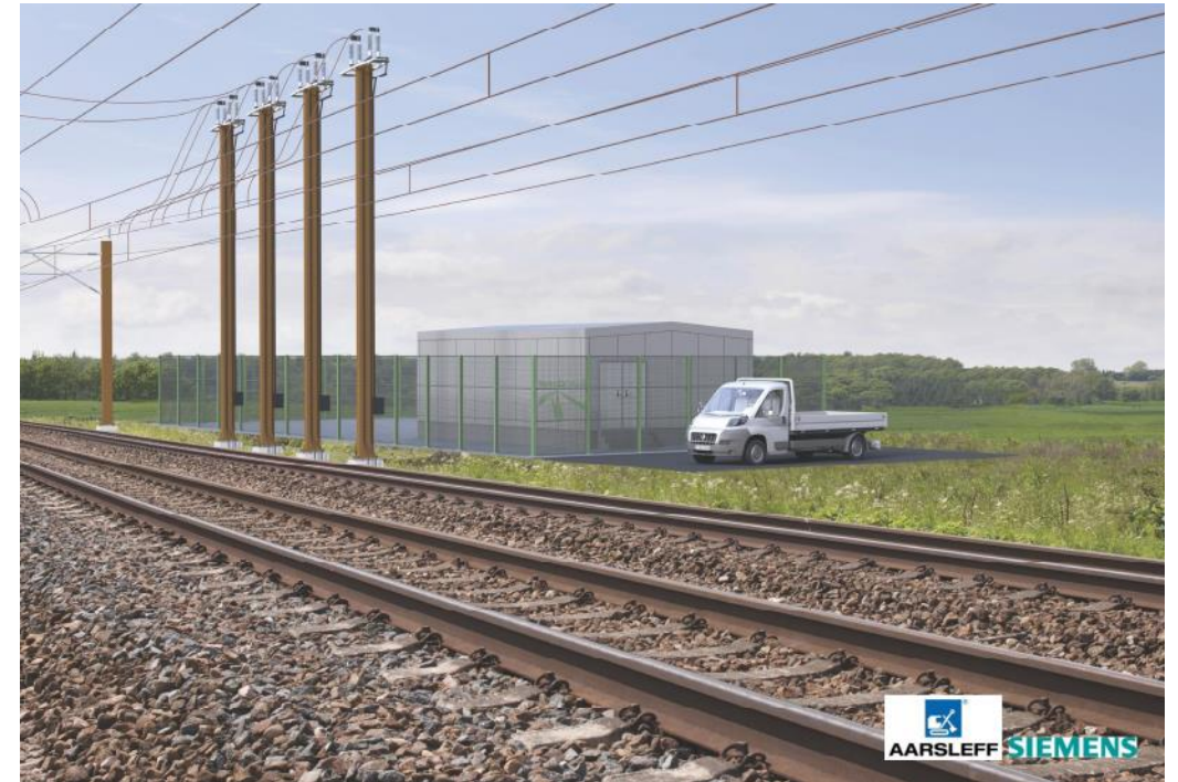
Autotransformerstation
